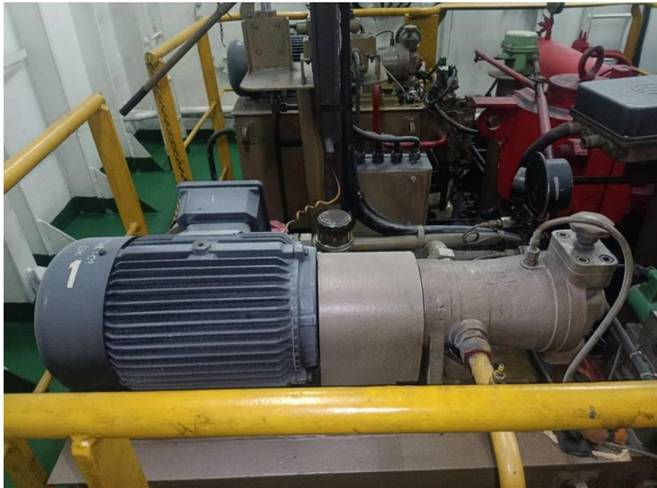
***Electric Motor Steering Gear***
