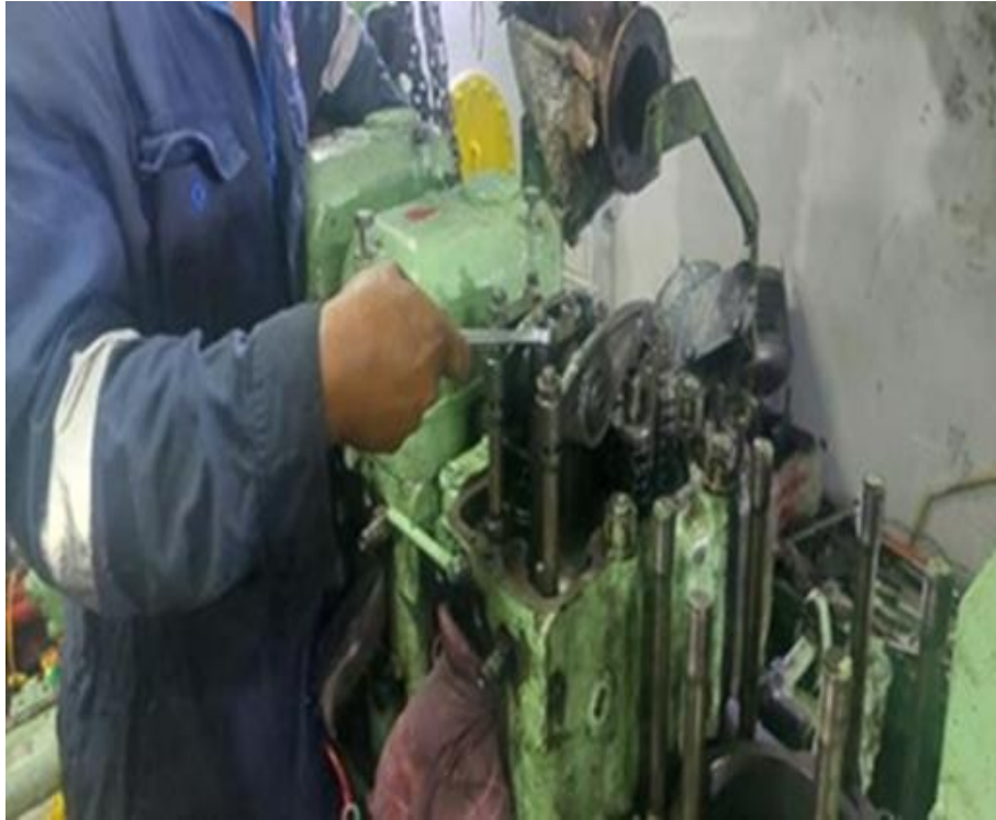
Lampiran C 11 Lepas Cylinder Head
