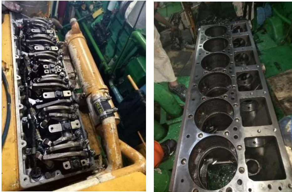
Gambar 3.3 Top Overhaul cylinder head AE 1 MT. Sea Reliance
