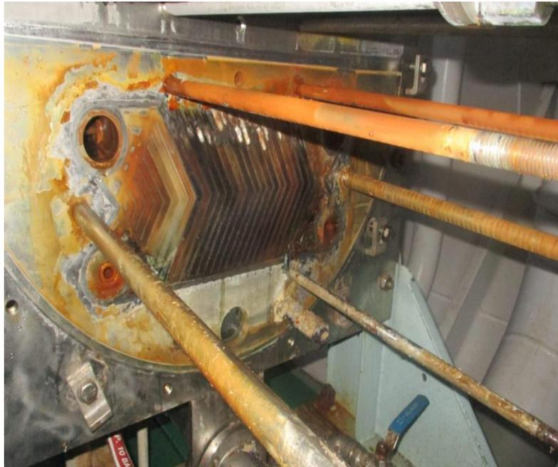
Gambar : Proses Pembersihan Fresh Water Generator
