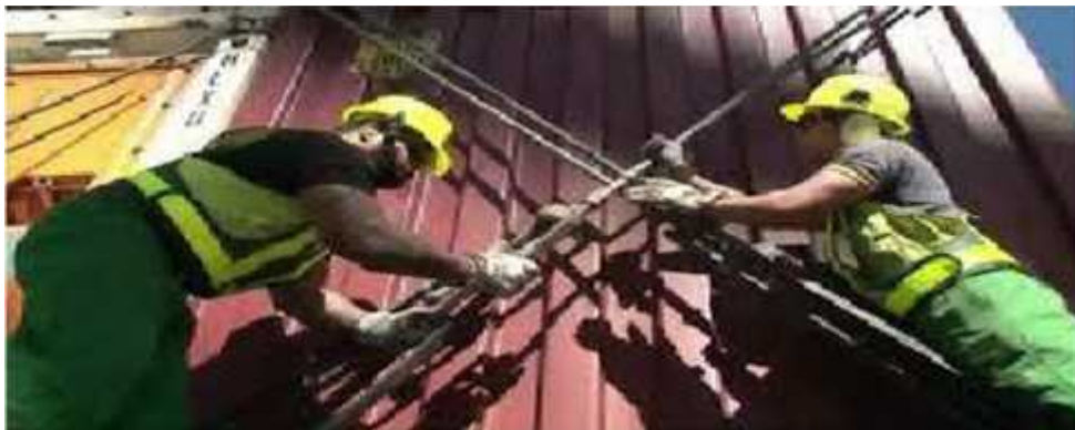
Gambar 2.2: pengecekan lashing bar and turnbuckle
