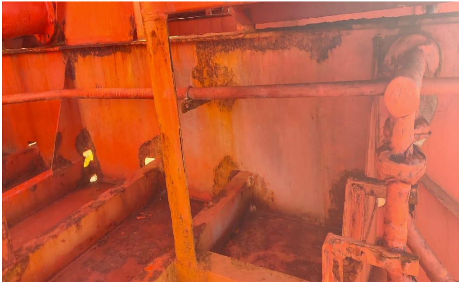
Gambar 2.5 Pitting Corrosion
