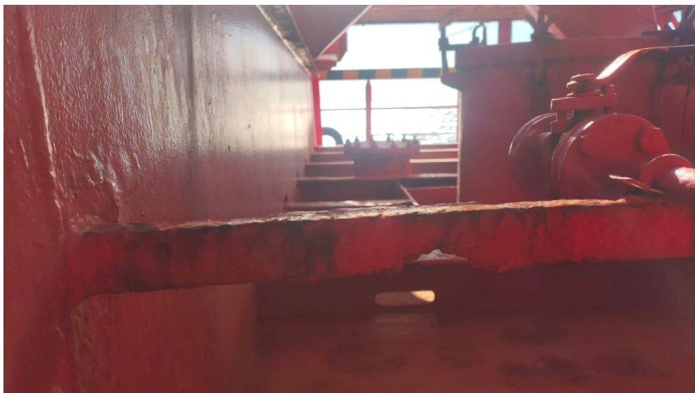
Gambar 2.4 Crevice Corrosion
