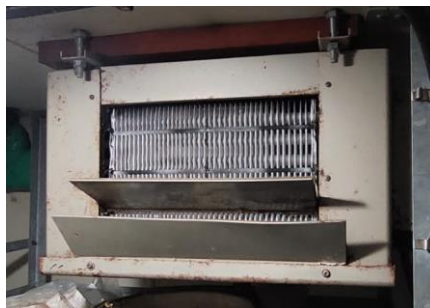
Gambar 2.3. Evaporator
