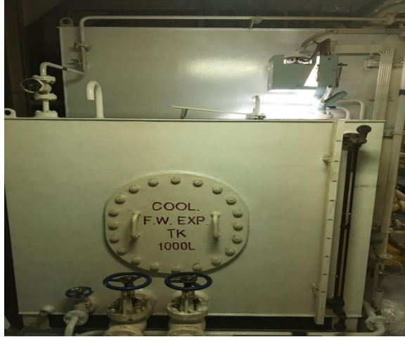
Gambar 4. 3 Fresh water expansion tank MT. Aspire
