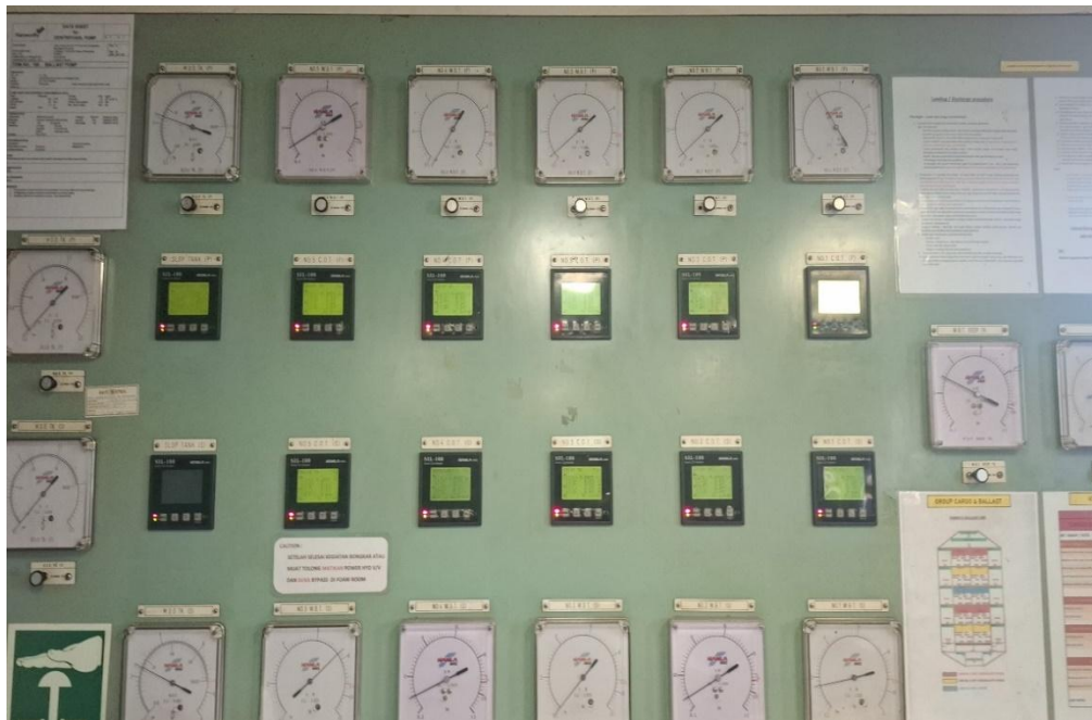
Gambar 2.7 Tank Gauging System
