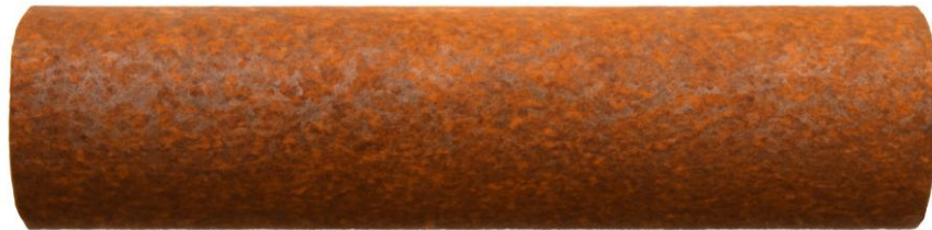
Gambar 2. 1 pipa korosi merata
