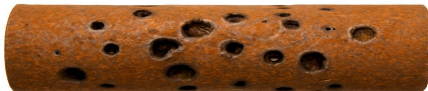
Gambar 2. 2 pipa korosi galvanik
