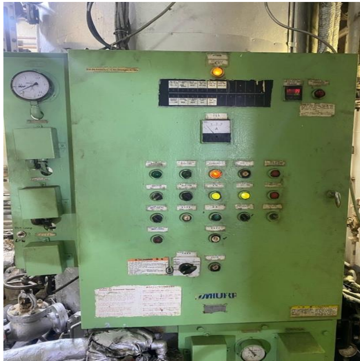
Gambar 2. 6 Panel Boiler
