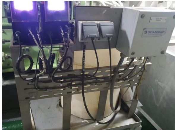
Gambar 2.9 Defoamer/Anti Foam Dosing Unit .
