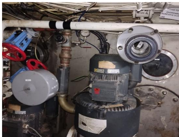
Gambar 2.8 Bioreactor Blowers
