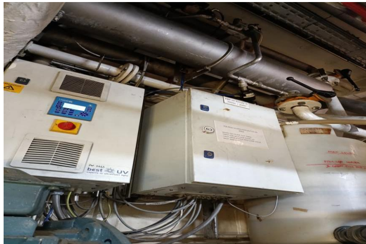
Gambar 2.16 Disinfection Unit (UV Chamber)
