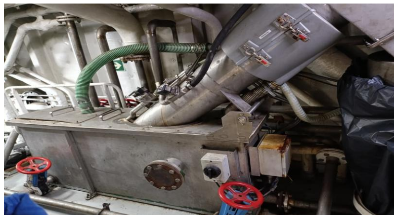
Gambar 2.6 Screening/Pretreatment Unit
