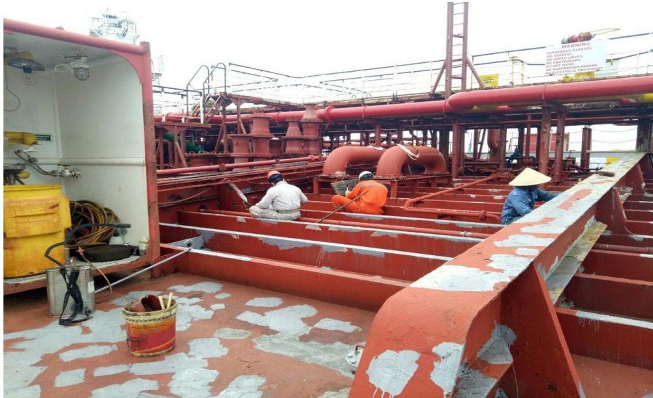
Gambar 4.4 Crew Deck Maintenance
