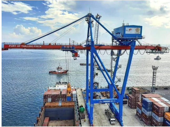
Gambar 2. 1. Quay Container Crane (QCC)
