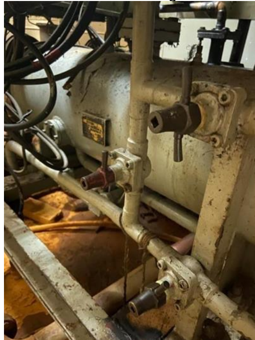
Gambar 4.5 Valve Pengisian Freon
