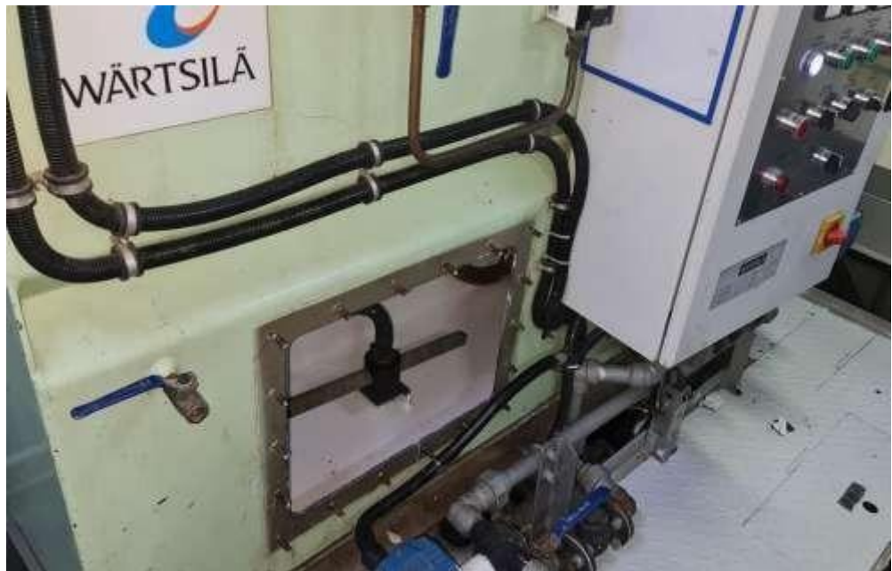
Gambar 3. Aerator/diffuser
