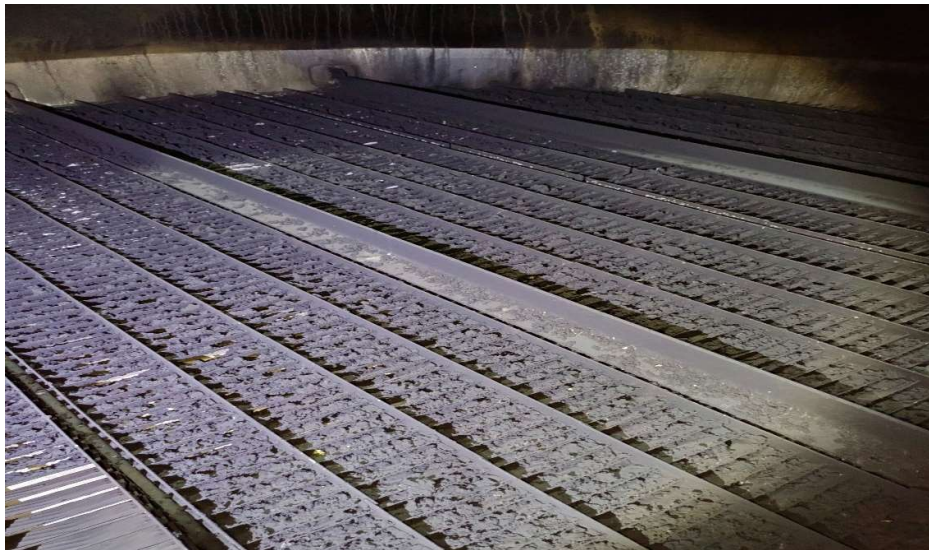
Gambar 2.9 : Mist Eliminator (dirty condition)
