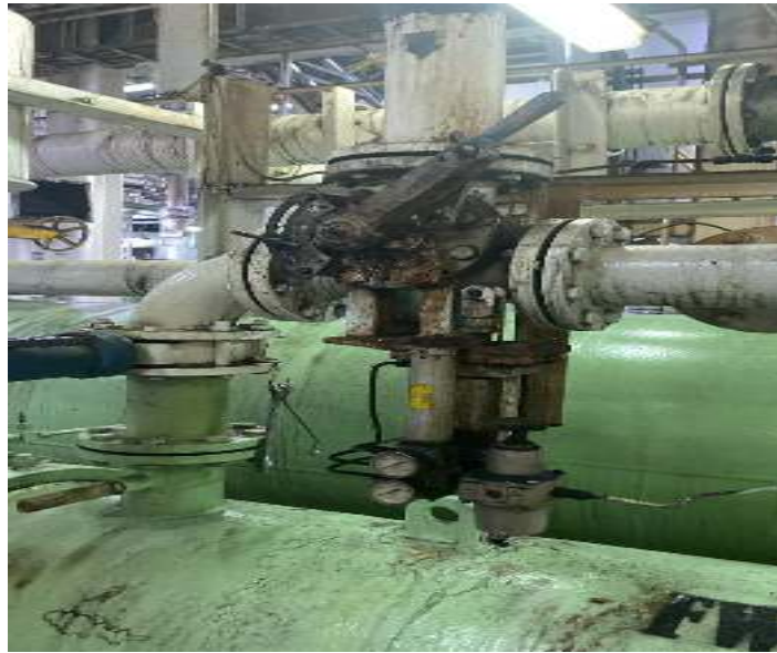
Gambar. 3.1 Three way valve
