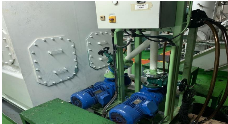
Gambar 2. 5 Vacuum pump .
