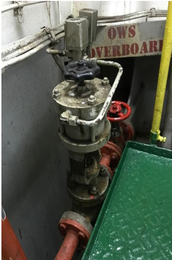
Gambar 2.6. Solenoid Valve
