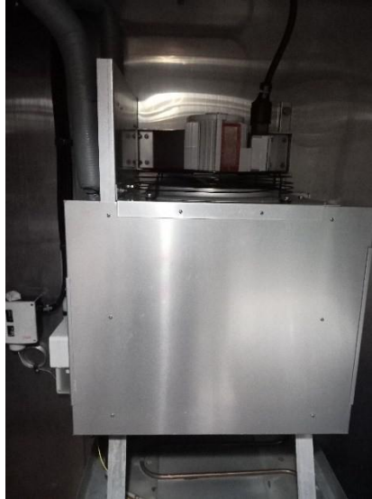
Gambar 2. 2 Evaporator
