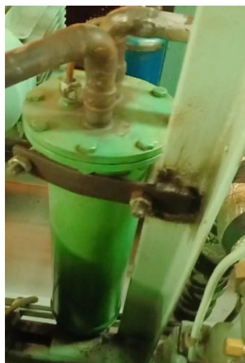
Gambar 2. 4 Oil separator
