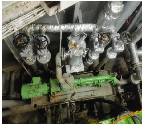
Gambar 2.6 Screw Pump
